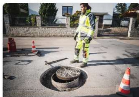
4. Removing the hatch
