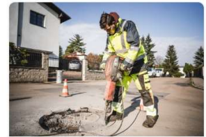
3. Demolition around the existing frame
