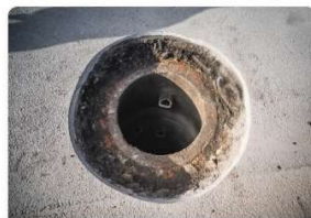
5. Cleaning the hole
