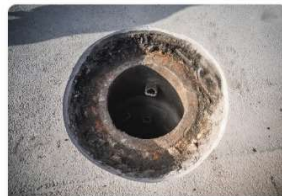
5. Cleaning the hole
