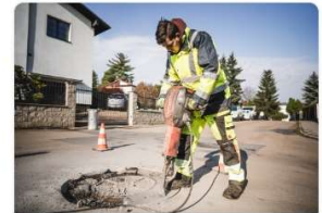
3. Demolition around the existing frame
