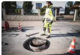
4. Removing the hatch
